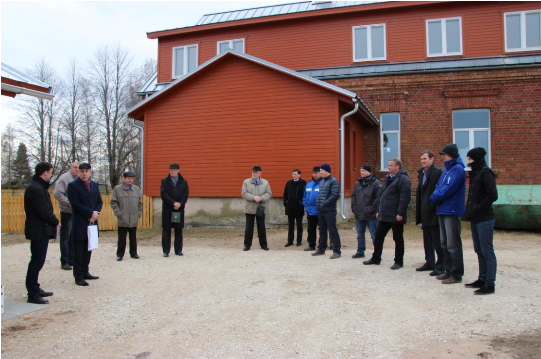
Photo 9. Ceremonial opening of newly constructed water treatment plant in Tiheda village, Kasepää Municipality
