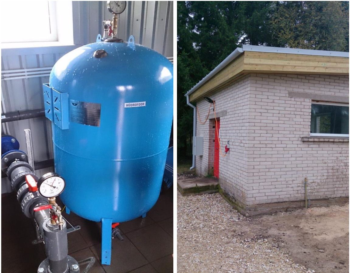
Photo 10 and photo 11. Constructed water treatment plant in Kükita village
