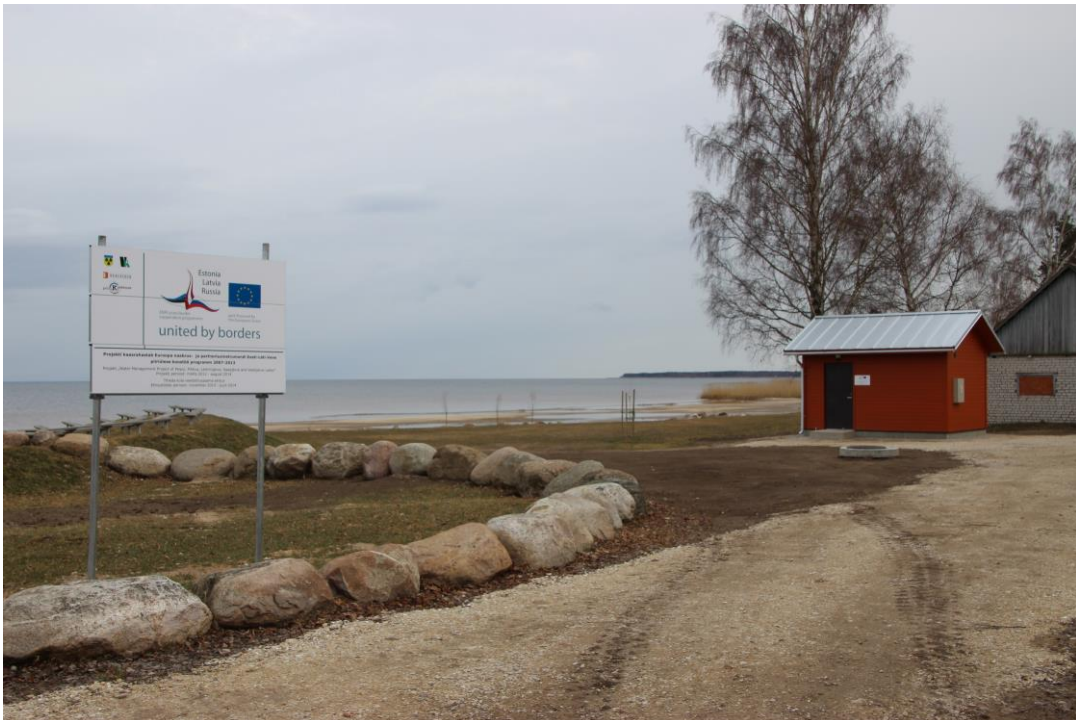
Photo 10. Constructed water treatment plant in Tiheda village, Kasepää Municipality
