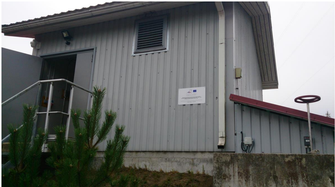
Photo 3. Mustvee wastewater treatment plant
